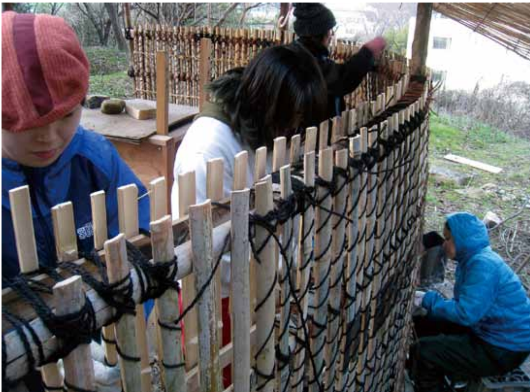
↑ Normal post-and-beam construction with one layer bamboo lattice
